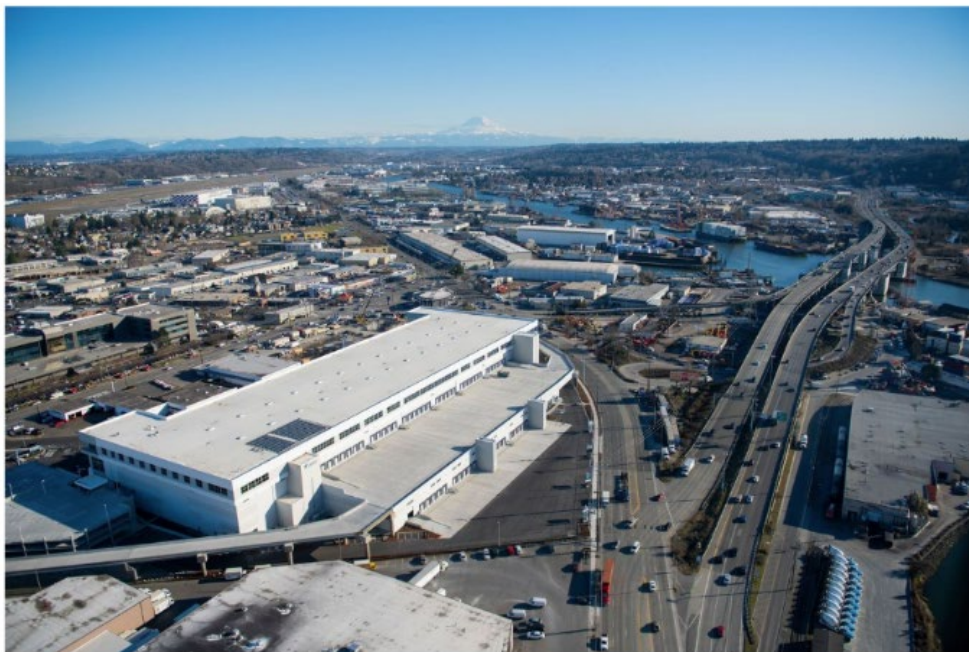
Prologis Georgetown Crossroads, a three-floor 590,000 square-foot industrial warehouse in Seattle. PHOTO: WOODY WELCH/PROLOGIS
